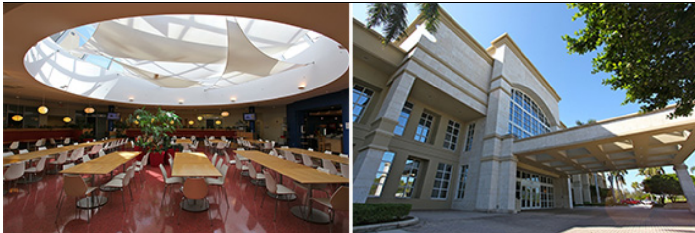
2100 West Cypress Creek Road in Fort Lauderdale
